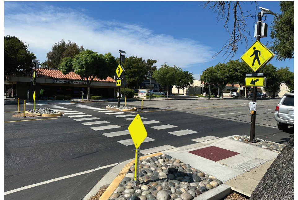
Mid-block crossings and pedestrian refuges make walking safer and more comfortable for pedestrians
